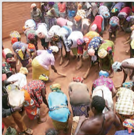
Making a floor using local clay
